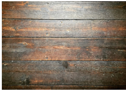
Original Historic Wood Flooring
